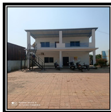
Fig. 4.3 Shankar Talav Village Panchayat office
