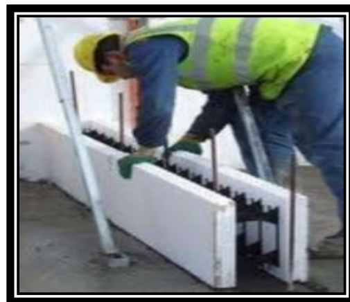
Fig. 14.10 Insulating Concrete Formwork
