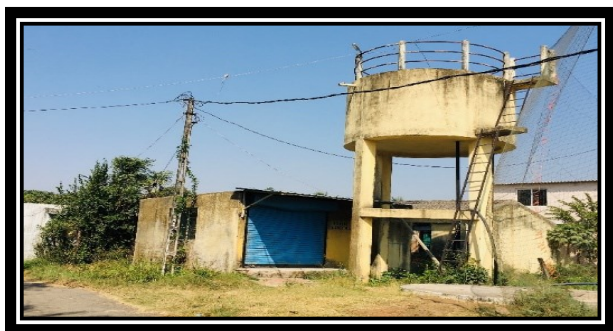
Fig. 4.14 Water Tank of Shankar Talav
