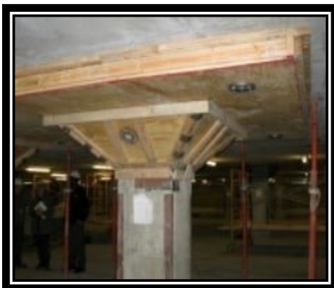
Fig. 14.7 Flat slab Construction
