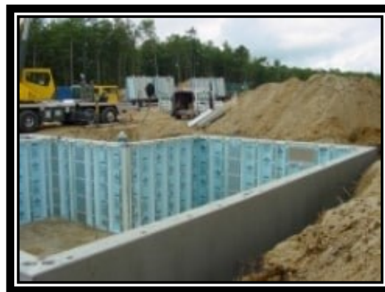
Fig. 14.8 Precast Concrete Foundation
