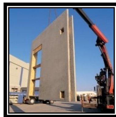
Fig. 14.5 Precast flat panel system
