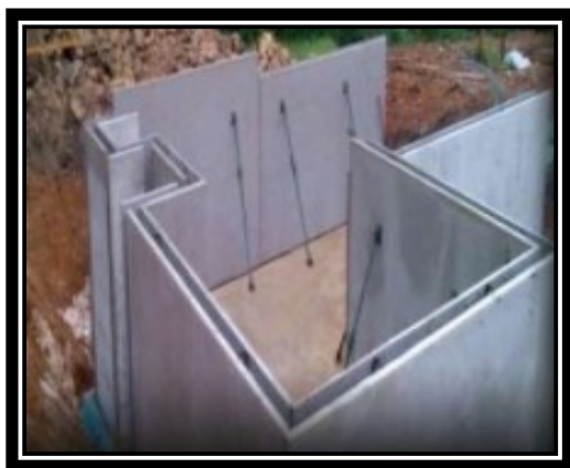
Fig. 14.9 Twin Wall Technology units are placed in the site.
