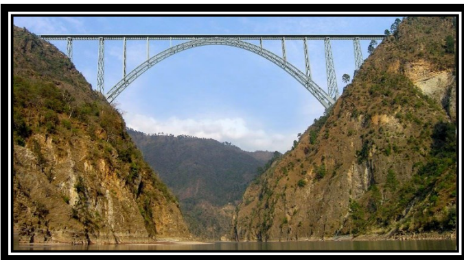
Fig. 5.12 Rail bridge over chenab river
