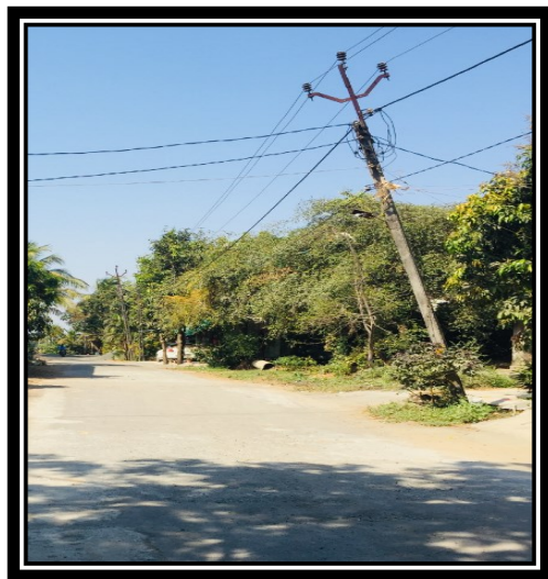
Fig. 4.23 Electric poles (Shankar Talav)
